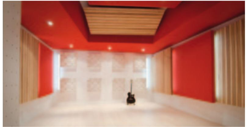
Figure 10. CDM Productions, Switzerland. Finished recording room with diffusors, ceiling and wall absorbers.
